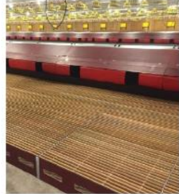
The barn now includes hardwood slats with galvanized slat supports.
